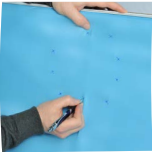
Locate and mark the position of the screws
